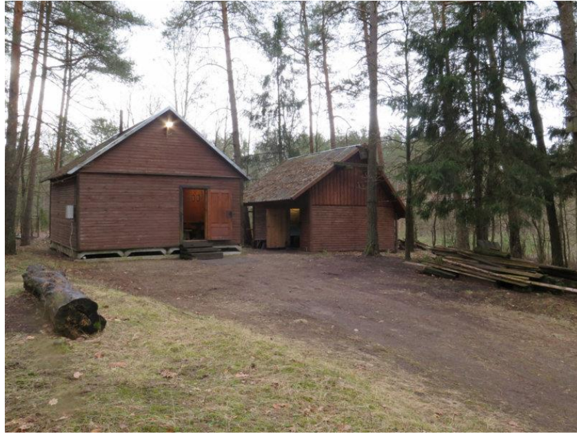
Figure 35 : hunting lodge with a separate dressing and storage room (right)
